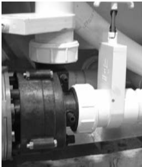
Slice Valve and Pump Union
