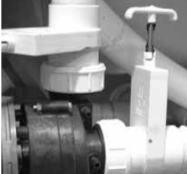
Slice Valve and Pump Union
