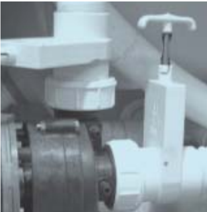
Slice Valve and Pump Union
